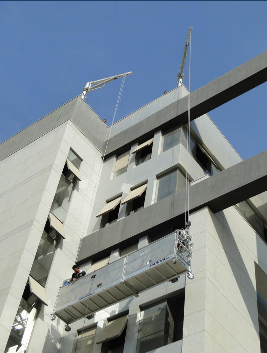
3 and 5 m mesh cladded Light Weight Stage for permanent installation with Alpha 500 hoists, Sky Locks, wire winders and rotatable davit arms.
