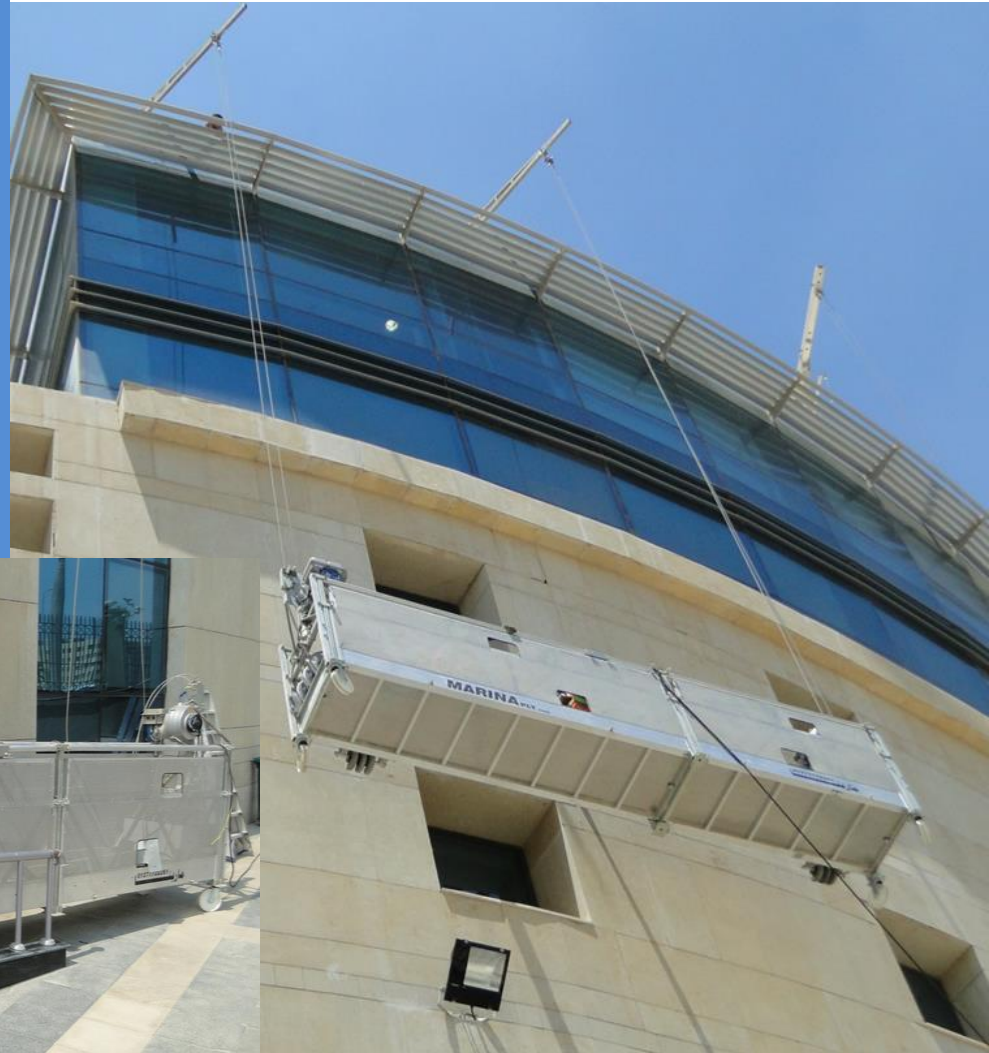
5 m mesh cladded LWS PI with Alpha 500 hoists, Sky Grips and access ladder
